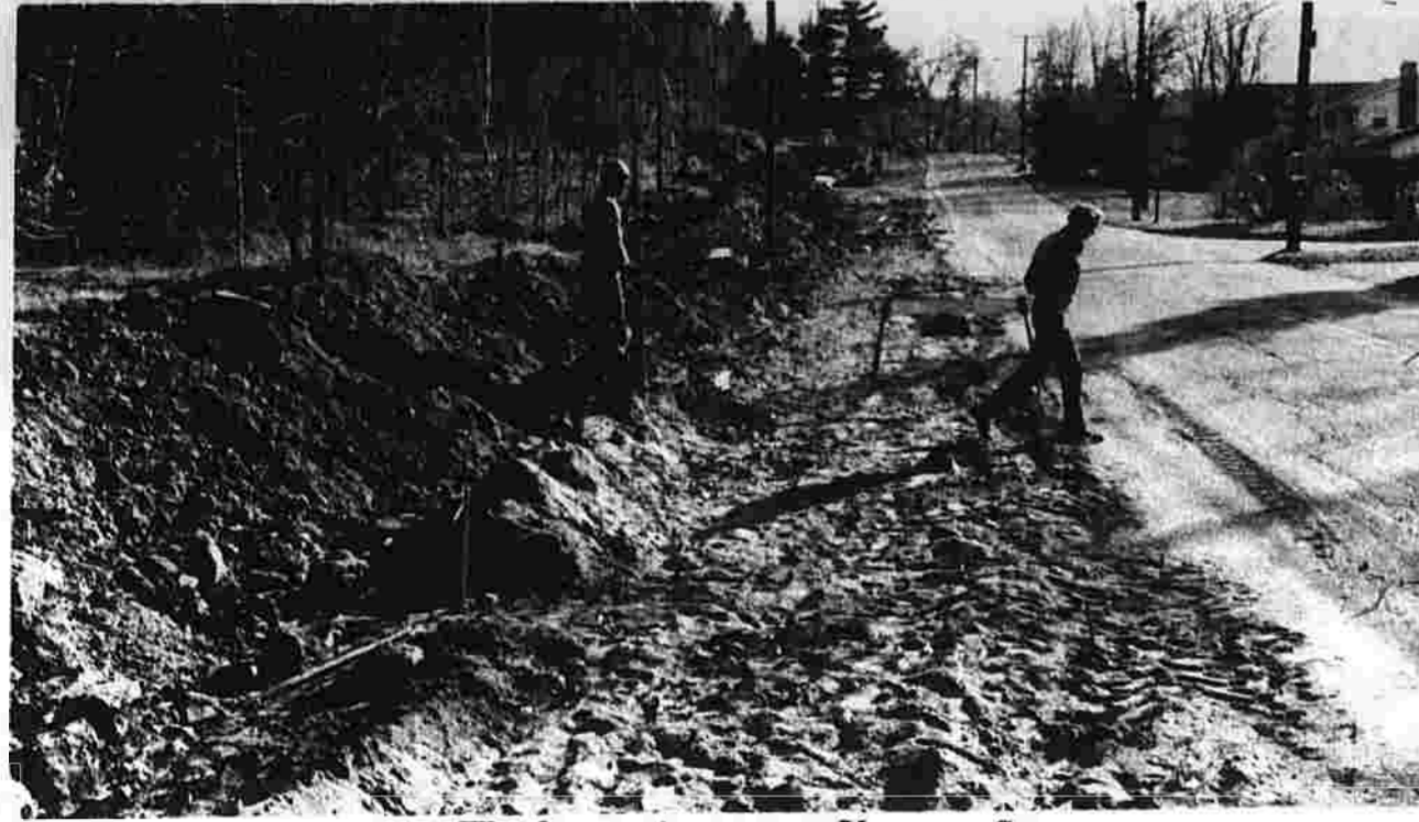
Work continues on Vernon Street
